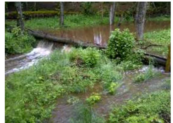
**Timber minibunds observed to be working but still to be tested under extreme events (potential to store several thousand m<sup>3</sup> of flood water).**
