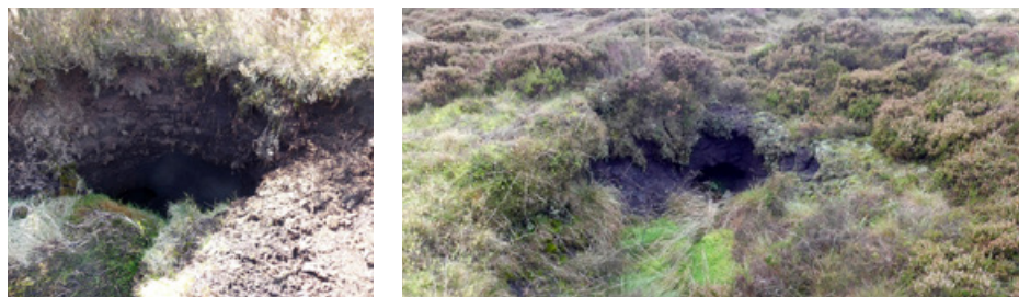
Fig. 2. Photographs of collapsed sections along large, deep mineral-based pipes at Arnfield (photo by A. West-Samuel).
