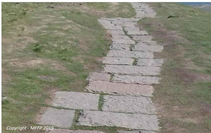
Figure 1: example of flagstones path, on an already restored section of the Great Ridge.
