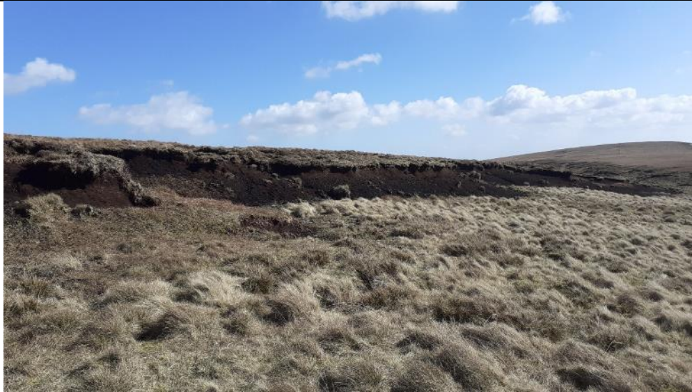
Photo 1 Photo showing typical bare peat hagg edge identified for re-profiling.
