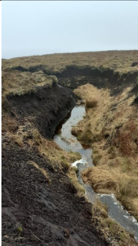
Photo 2 Photo showing typical location for stone dam; here a two unit stone dam has been proposed due to the width, height and potential sediment load of the gully. The gully sides shown here are approximately 2.25m in height and will also be subject to re-profiling and subsequent bare peat revegetation techniques
