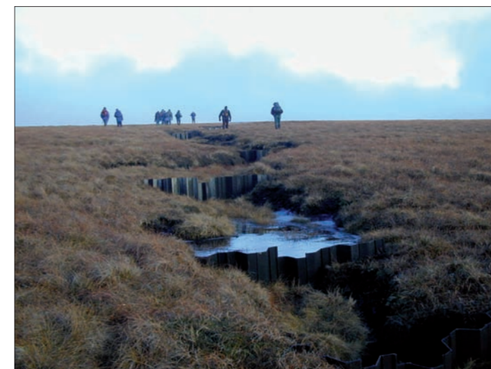
Pools form behind plastic gully blocks on Within Clough
