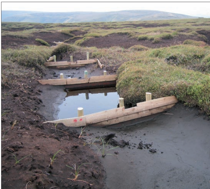
Wooden fence gully blocks
