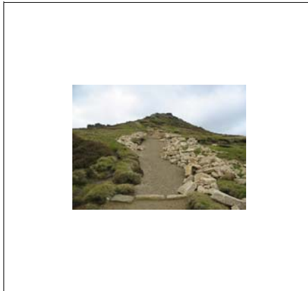
Path restoration work underway on Higger Tor
