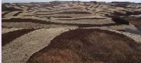
Geo-textiles used to stabilise peat slope
